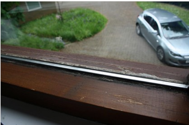
Internal 1st floor window
