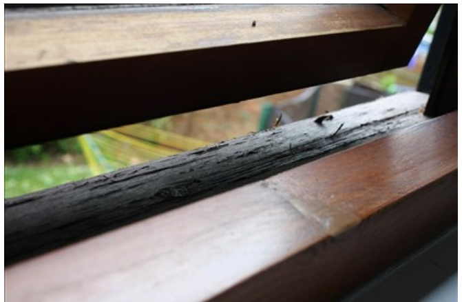
External & Internal 1st floor window
