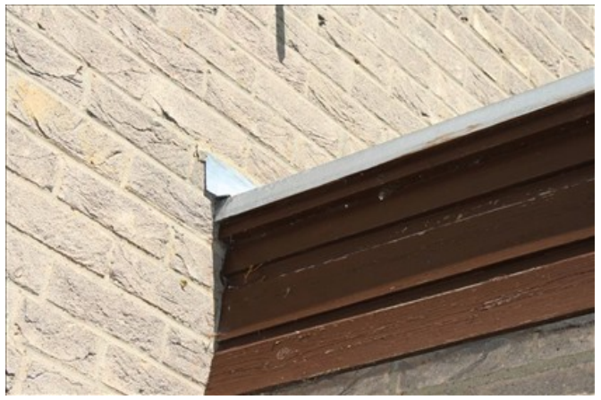
Timber board to edge of flat roof
